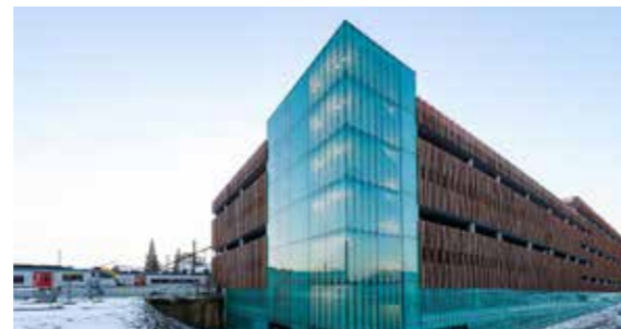
KAAI DISTRICT, AALST, BELGIUM
