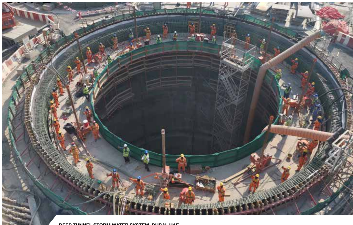
DEEP TUNNEL STORM WATER SYSTEM, DUBAI, UAE
